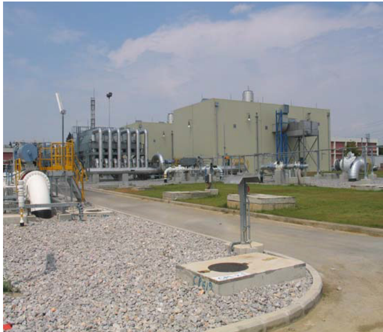
Picture 1: Compressor Station at Nea Mesimvria, Thessaloniki
