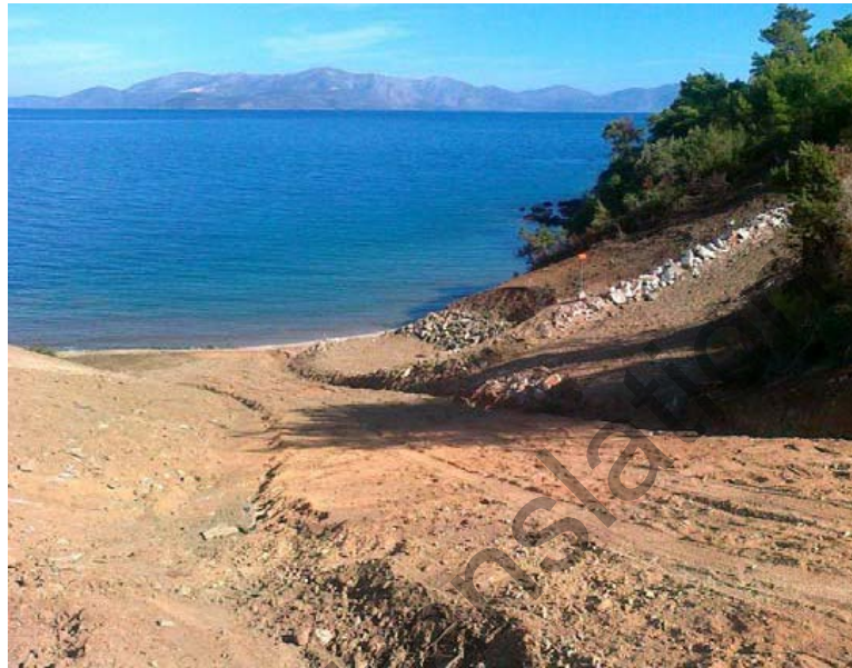
○ ○ Picture 1: Routing of the pipeline to the underwater section of Aliveri branch
