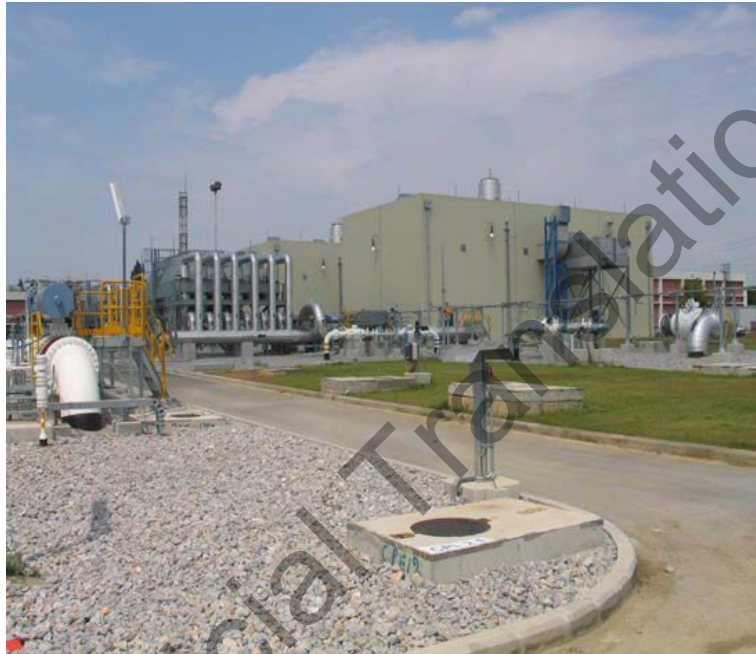
Picture 2: Compressor Station at Nea Mesimvria, Thessaloniki
