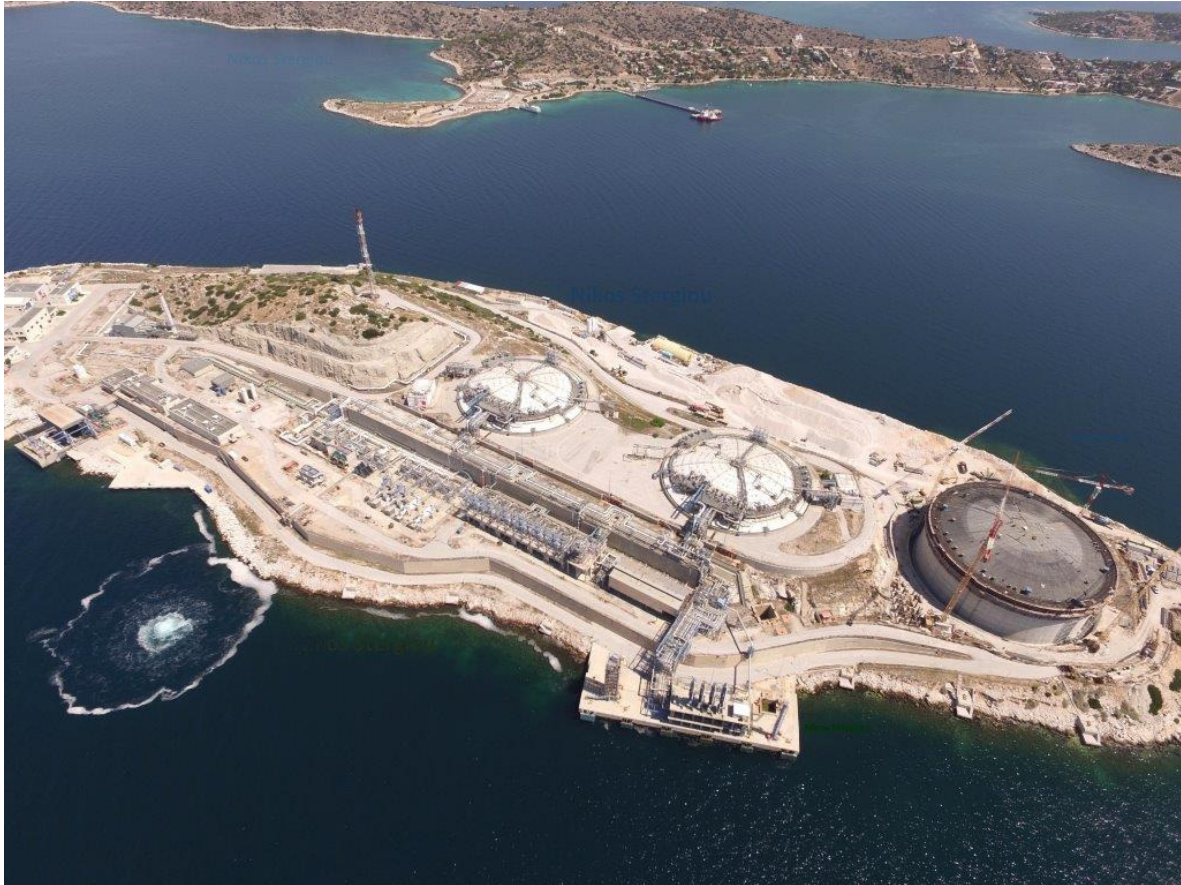
Picture 2: Aerial view of terminal station with the installation of the 3rd tank
