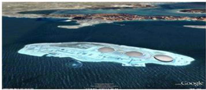
Picture 1: Aerial view of terminal station with the installation of the 3rd tank
